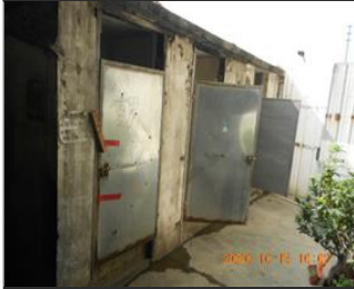
Photo of the sanitary facilities Toilet.JPG
