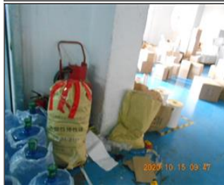
Photo of non-conformity NC Blocked fire extinguishers.JPG
