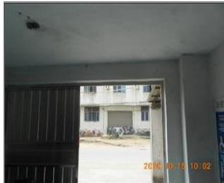
Photo of non-conformity NC No exit sign or emergency light for safety exit 1.JPG
