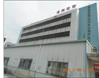
External photo(s) of the production unit(s) Production and warehouse buildings.JPG
